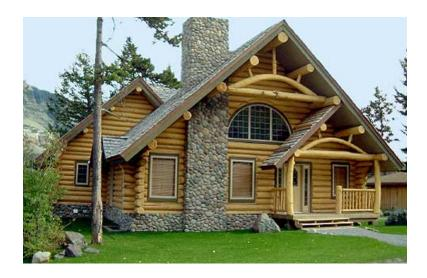
Machine-made logs usually have no taper, are a more uniform size and have even joinery in the corners.
